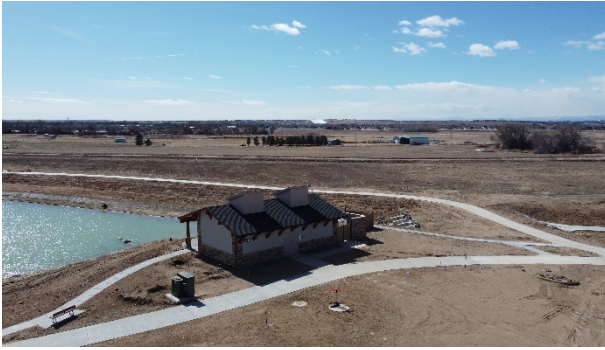
Non-Potable Pumpouse View: Southwest
