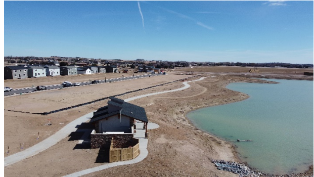
Non-Potable Pumpouse View: Northeast
