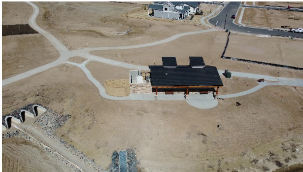
Non-Potable Pumpouse View: Northwest
