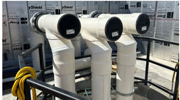
Pumphouse View: Ground
