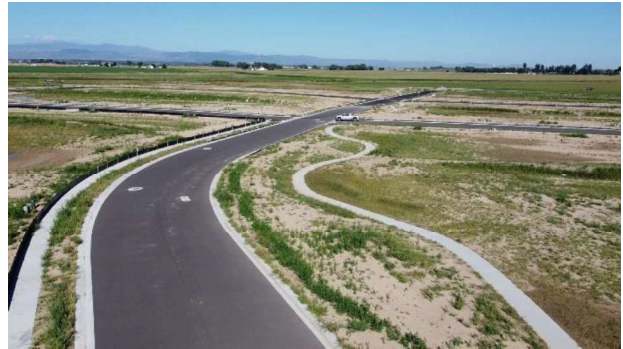
Kettlepond Rd from Rhapsody Drive View: Northwest
