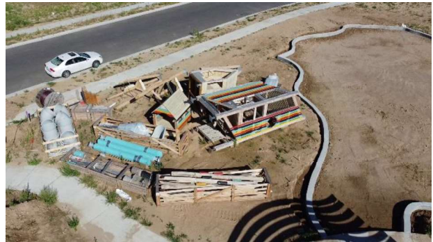
Playground Stored Materials View: Northwest
